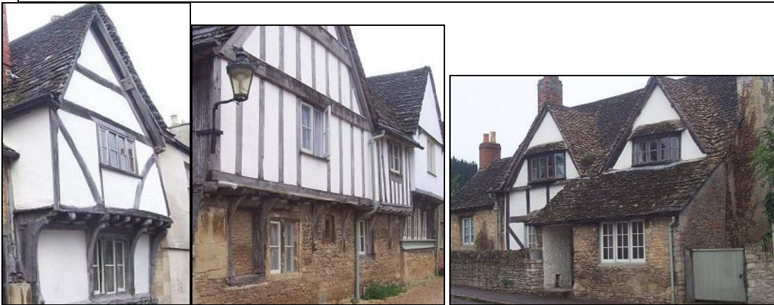
1. 2. 3. 4. Timber houses in Lacock (England).
